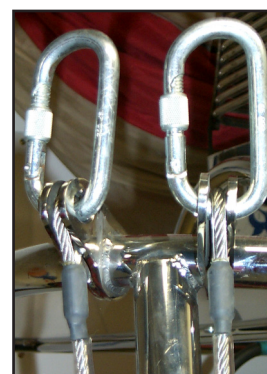
▲ Rigging Of Frame Type 'D'
