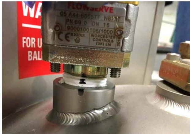
Figure 1 - Alignment marking on thread and boss
