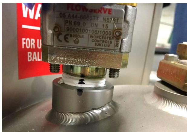
Figure 1 - Alignment marking on thread and boss
