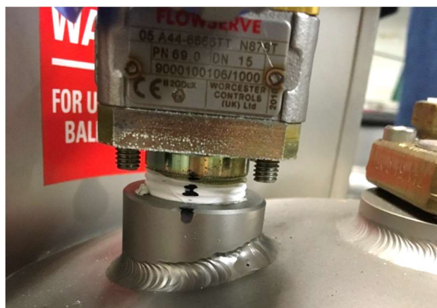
Figure 1 - Alignment marking on thread and boss
