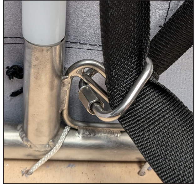
▲ Harness bottom frame attachment
